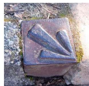
Alignment Pin references road alignment
