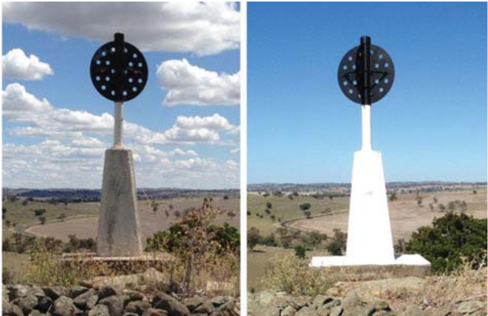
Figure 4: TS6603 Nimby before and after trig maintenance.
