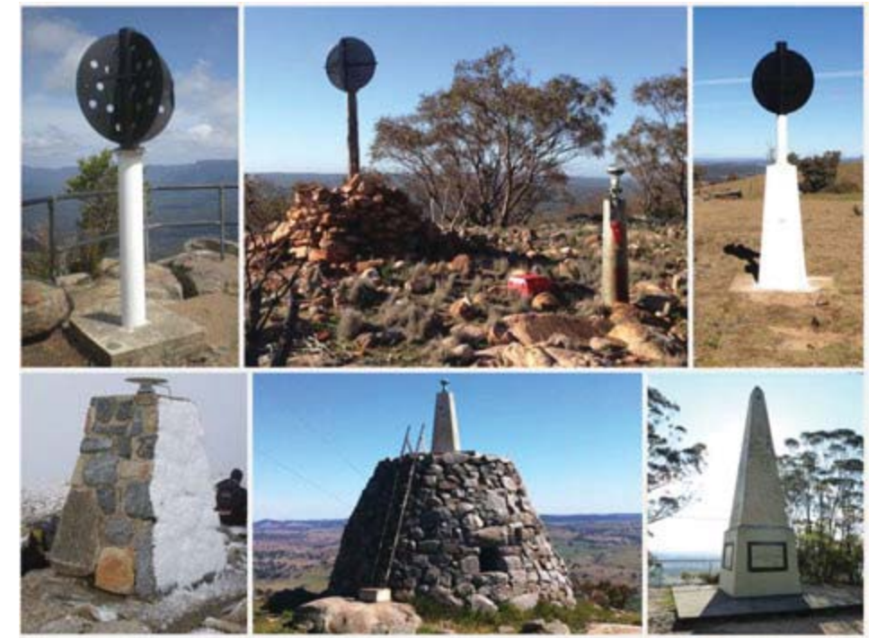
Figure 2: Trig station monuments in NSW. Clockwise from top left: Steel pillar, cairn and astro pillar, concrete pillar, obelisk, concrete pillar on grand cairn, and stonework veneer on concrete pillar.
