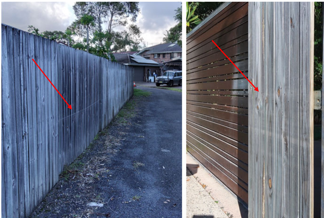
Figure 17: Scouring caused by debris moving past a structure.
