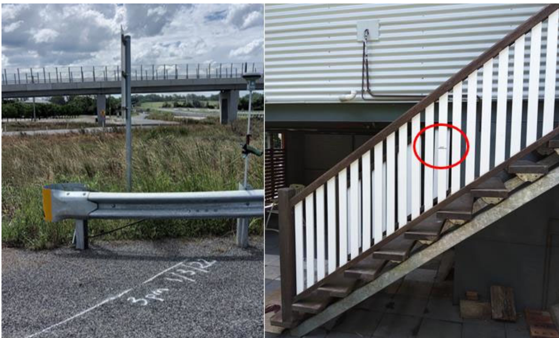
Figure 21: Marking provided by residents, volunteers and/or workers.
