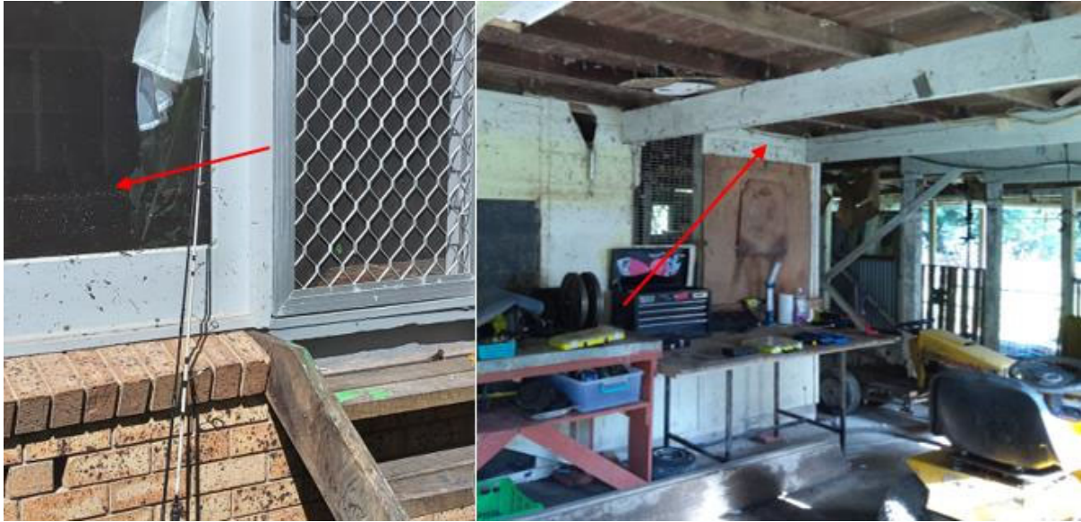
Figure 18: Small debris requiring horizontal offsets.
