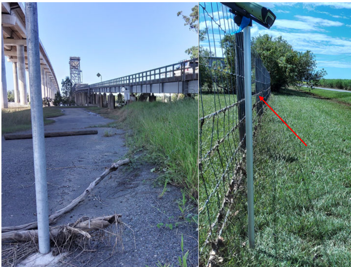
Figure 15: Large debris remains near rivers.
