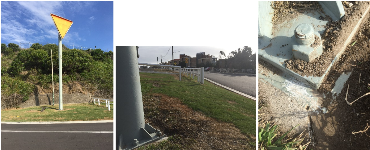
Figure 14: Recovery mark placed in concrete base of ship navigation target (CQ from DP).
