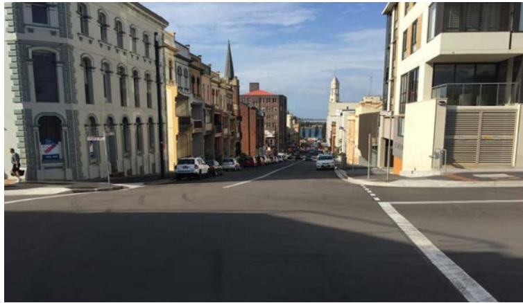
Figure 9: Looking north down Watt Street to the foreshore of the completed works (at the intersection of Shortland Esplanade).
