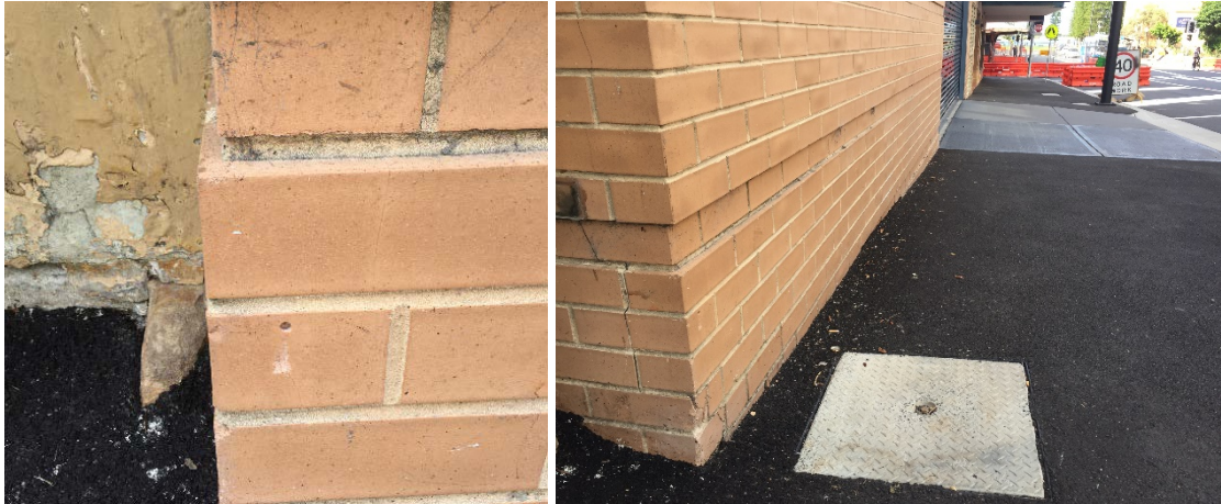
Figure 11: Recovery mark placed in wall (AO from DP).
