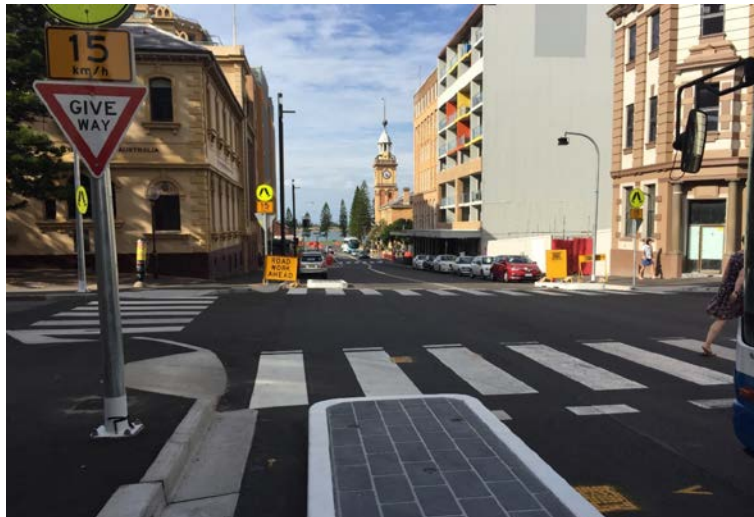
Figure 10: Looking north down Watt Street to the foreshore of the completed works (at the intersection of Hunter Street).
