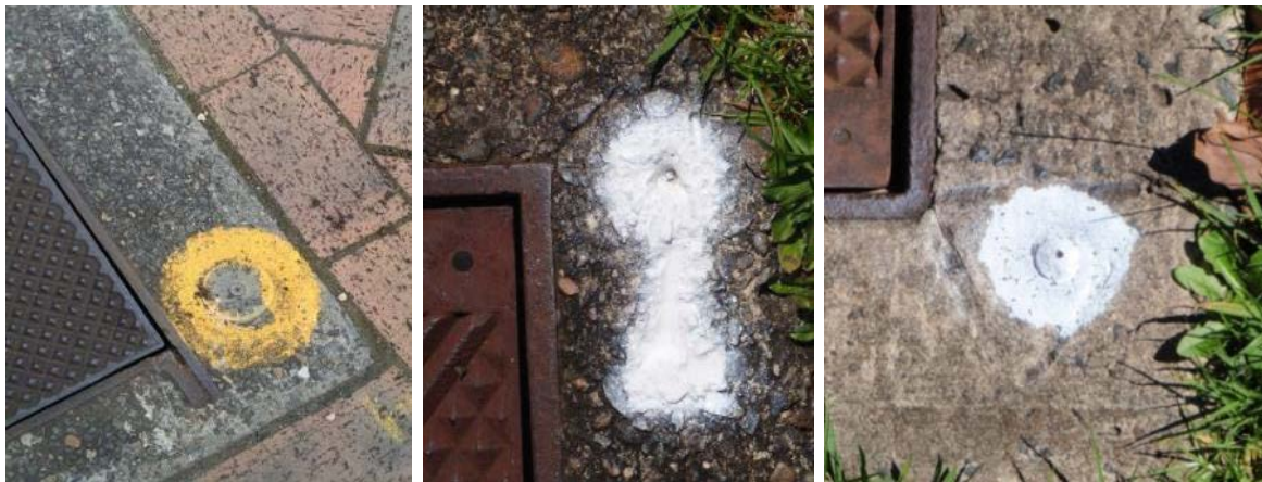
Figure 15: State Survey Mark in telco pit, reference mark in pit, and bench mark in pit (de Belin, 2015).
