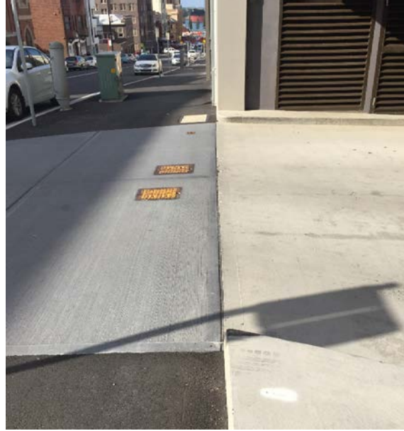
Figure 13: Recovery mark placed in concrete (FW from DP).
