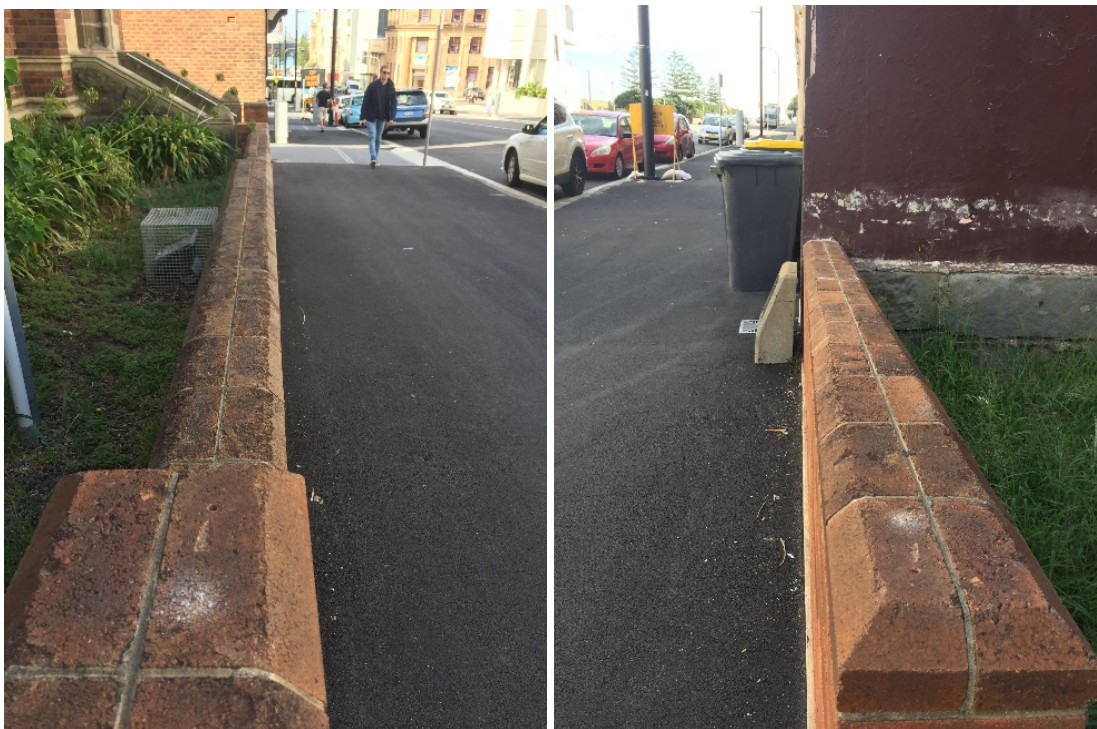
Figure 12: Recovery mark placed on top of brick wall (O from DP).
