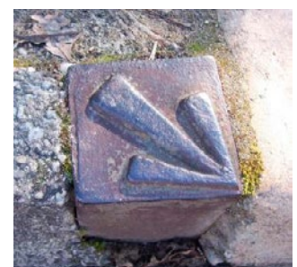
Alignment Pin references road alignment
