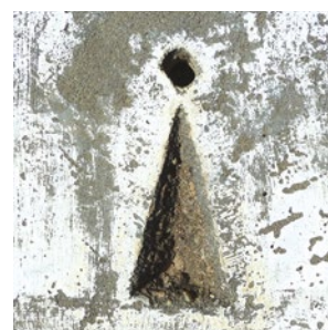
Drill Hole & Wing in Kerb references adjacent boundary corner
