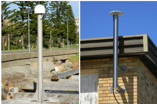
Figure 2: Free-standing pole and wall monuments at Tier 3 CORSnet-NSW sites.
