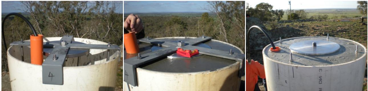
Figure 3: Construction of the GNSS CORS pillar plate at a Tier 2 CORSnet-NSW site.
