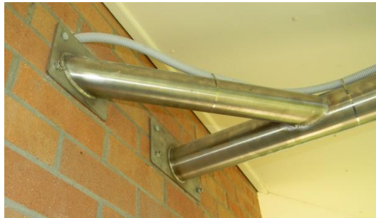
Figure 6: Using Anka screws (top) to hold the monument in position while the chemical anchors (bottom) cure at a CORSnet-NSW site (Tier 3).
