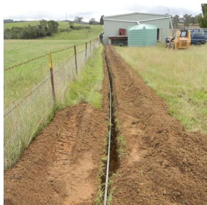
Figure 17: GNSS antenna cable and conduit being buried at a CORSnet-NSW site (Tier 3).
