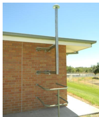
Figure 13: Handrail installed around the base of a CORSnet-NSW site (Tier 3).
