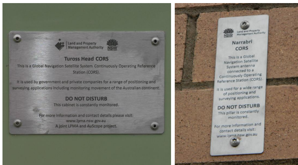
Figure 20: Monument inscriptions for Tuross Head CORS (Tier 2) and Narrabri CORS (Tier 3).
