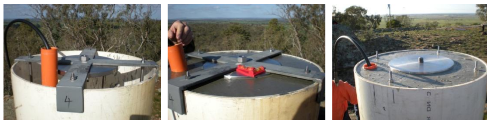
Figure 8: Construction of the GNSS CORS antenna mount at a CORSnet-NSW site (Tier 2).
