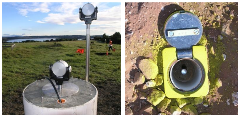
Figure 19: (a) RM survey being conducted during installation of a CORSnet-NSW site (Tier 2) before the GNSS antenna is installed, and (b) one of the reference marks placed for Tier 2 sites.
